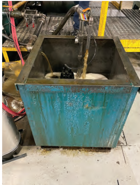
Shows improper mixing and evaporating
